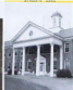
This is what the orphanage looked like before the fire-notice the belly on the roof.
